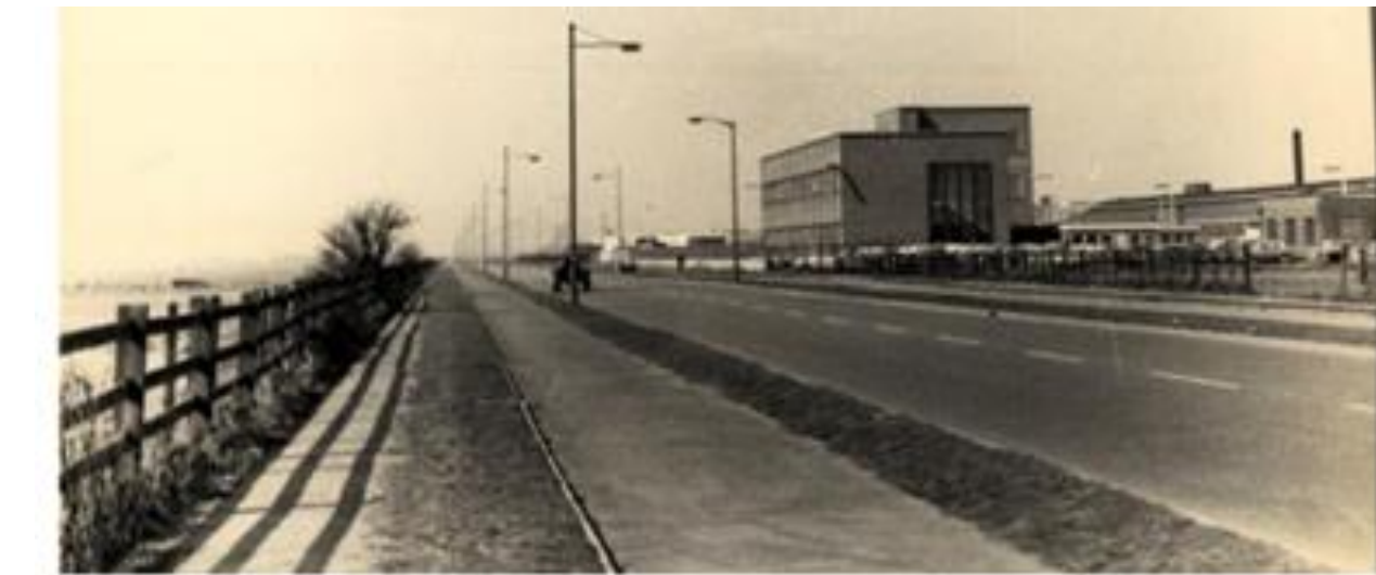
AEI building, Trafford Park, Manchester (1965): Although MV was acquired by Associated Electrical Industries Ltd (AEI) in 1928, the trading name was not changed until 1960. The AEI Scientific Apparatus Department was created and MV mass spectrometry research department at Trafford Park relocated to Barton Dock Road.
