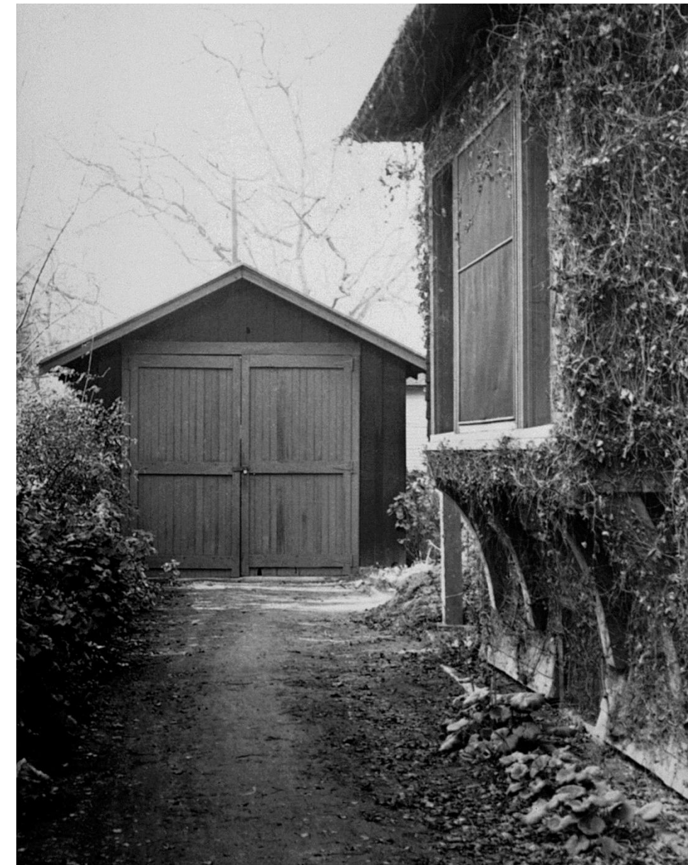
The garage at 367 Addison Avenue
